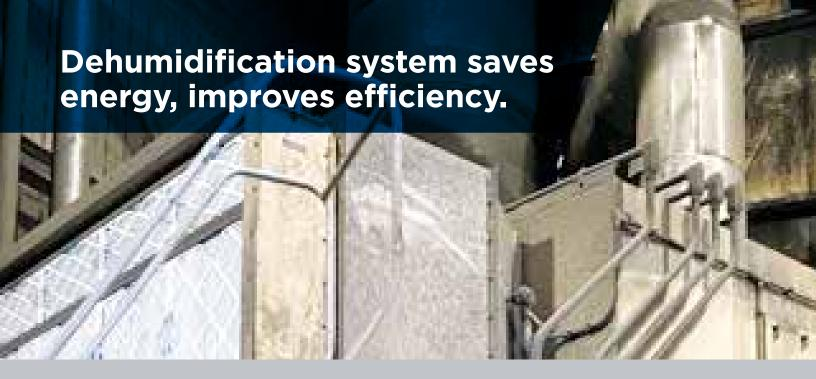
A revolutionary blast-air dehumidification system is decreasing energy costs, decreasing raw material use, and increasing melt efficiency.
