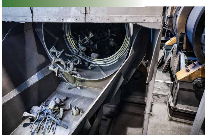
A new conveyor system at Plant 4 replaced a 30-year-old vibratory system in January 2024, reducing airborne dust and creating a healthier working environment.
